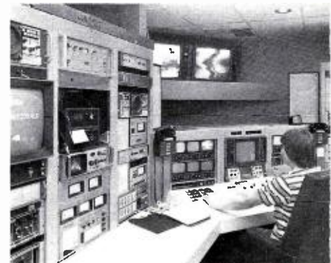
Master Control includes monitor displays of scrambled and unscrambled pictures.
