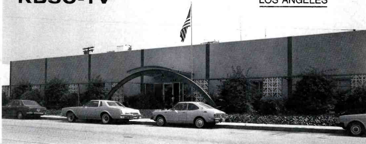
This Glendale facility is shared by KBSC-TV and National Subscription Television.
