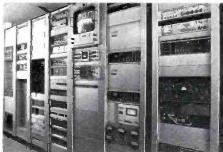
Master control console includes film camera shading controls; remote controls for film and tape "cart" machines, and multiplexers. Near Master Control are a bank of racks housing the TK-44 camera control units. Another row of racks mounts equipment for distribution, switching, monitoring and testing.
